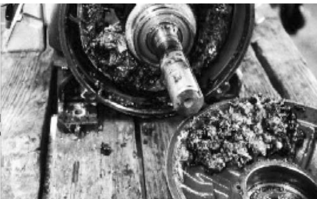
Figure 8. Overgreasing caused inside of motor to fill with grease.
