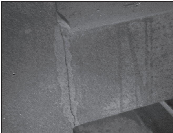
Figure 7. Frame Crack
