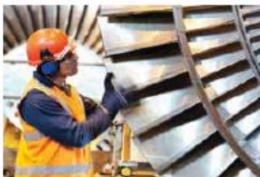
Industrial turbine systems
